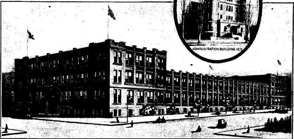
ADMINISTRATION AND INSTRUCTION BUILDINGS—I. C. S.
